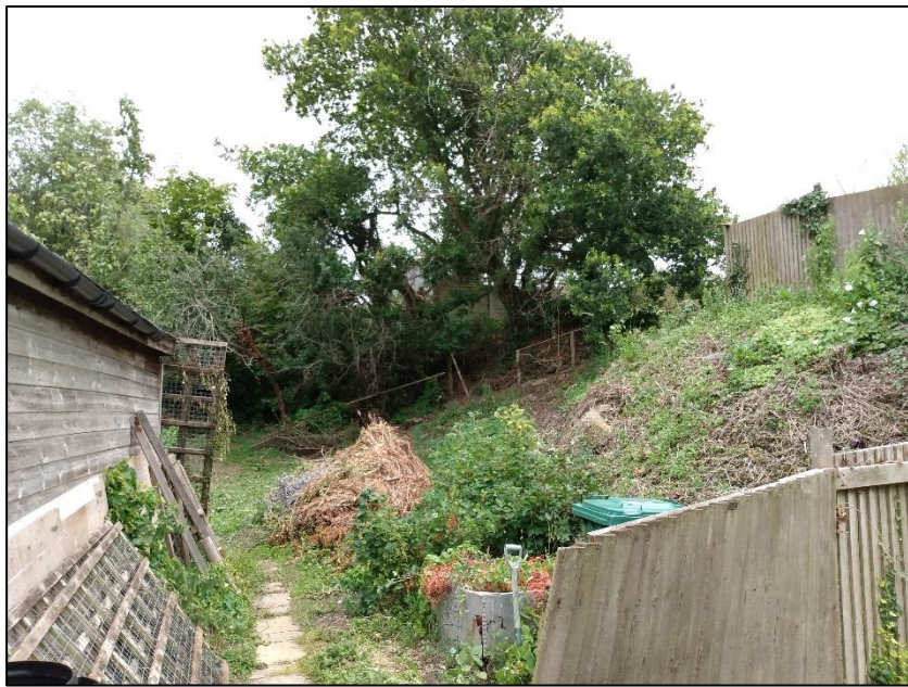
Facing east along southern flank of existing building
